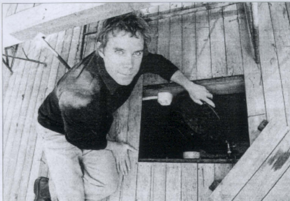
Luke Middleton installs a water tank.
