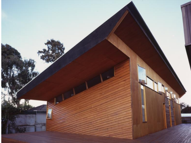
Figure 5: Thornbury High School general purpose classroom (Photographer: Scott Haskins)
