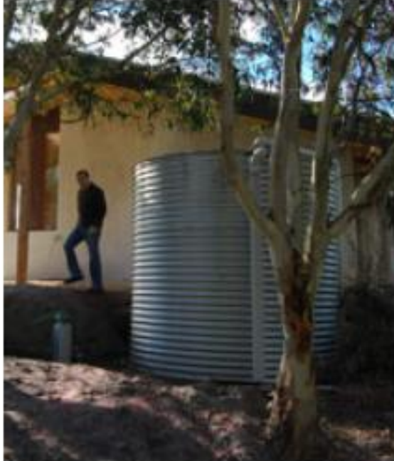
Figure 2: Rainwater tank, pump and recycled tyre retaining wall 11
