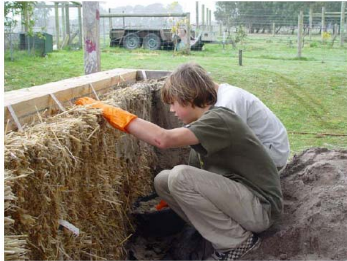
Figure 3 – Woodleigh students constructing the straw bale walls (Woodleigh School 2008)
