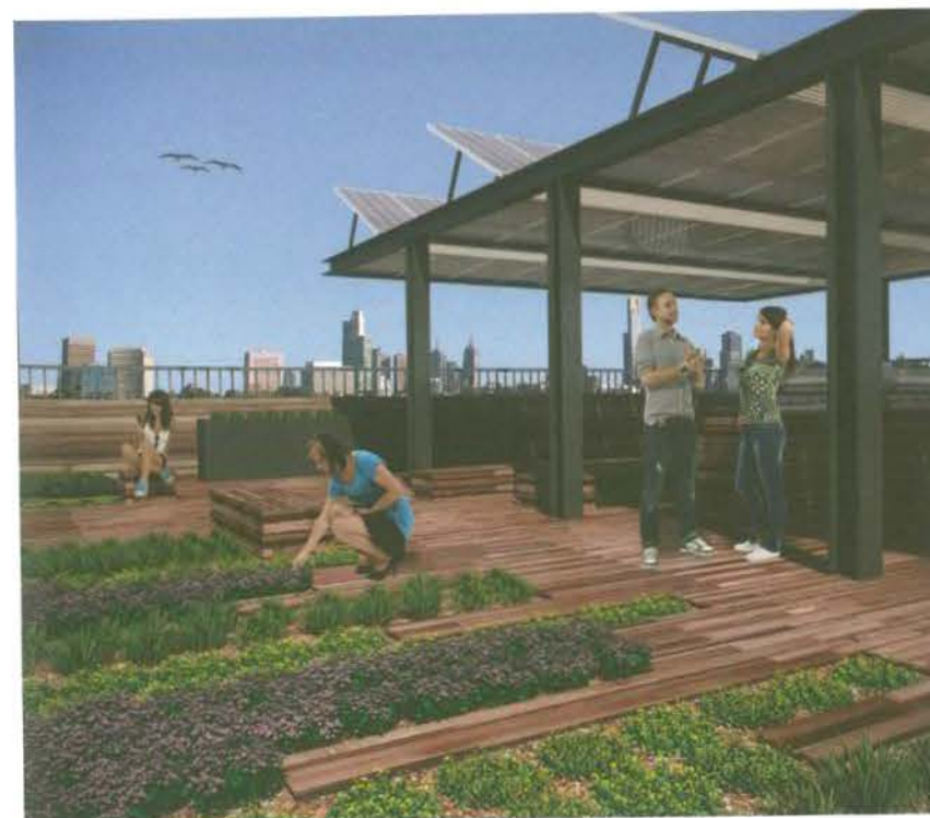
➤ The Commons rooftop garden will include a 5.9 kilowatt solar PV system and solar water heating system to service all apartments. All The Commons images courtesy Breathe Architecture
