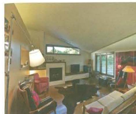
Louvred windows to the east enable breezes to circulate air throughout the apartment, and are shaded by the roof overhang to prevent harsh morning summer sun. "All of the apartments are designed so that you can open them up and get ventilation without feeling exposed," says designer Luke.
