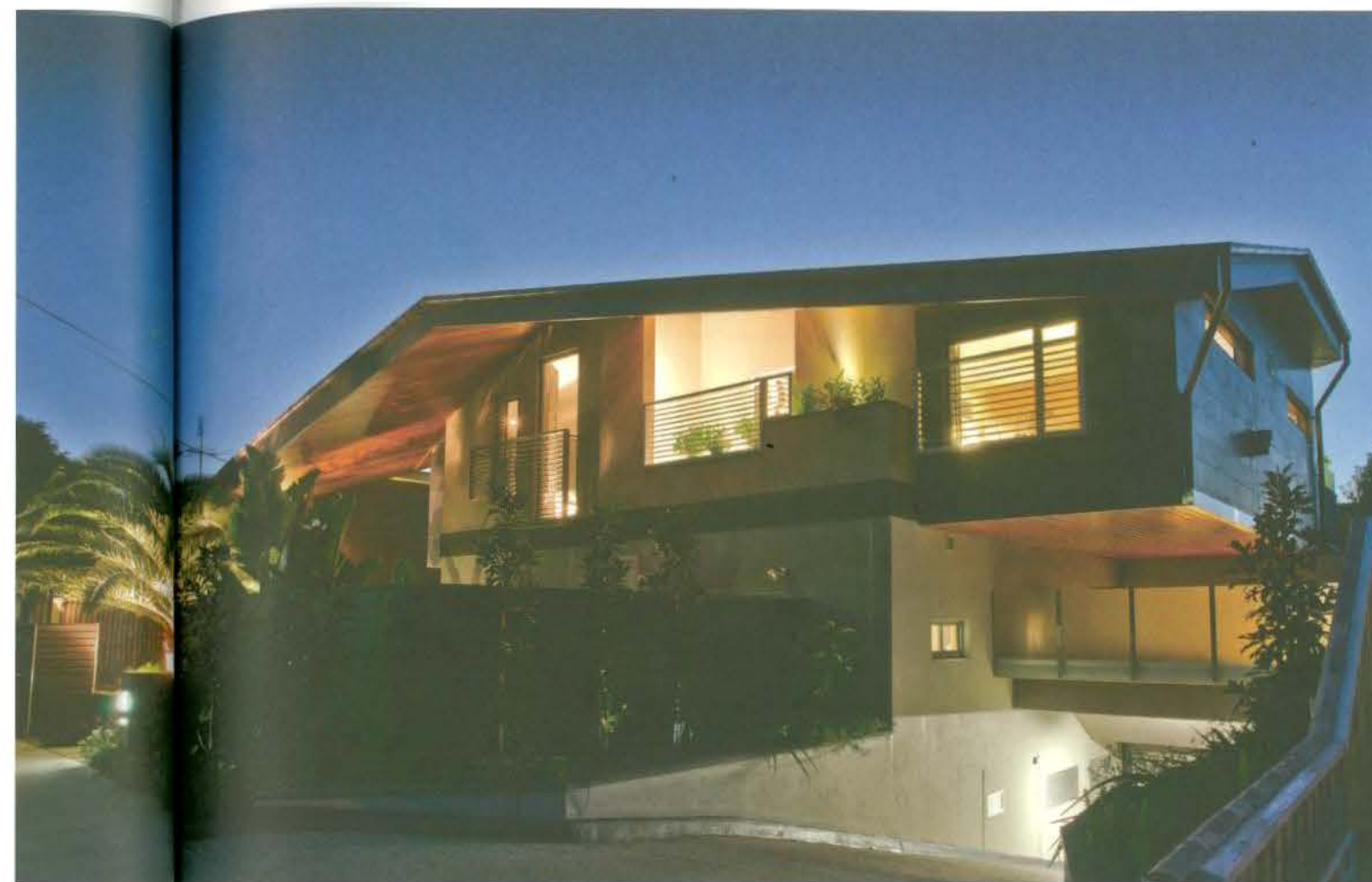
From the street, the Victoria Street Apartments look like one large home. Designer Luke Middleton from Eme Design based the roof's form on those of other houses in the area; it is also designed to let winter sun in, protect the homes from harsh summer sun and provide residents with entry protection.
