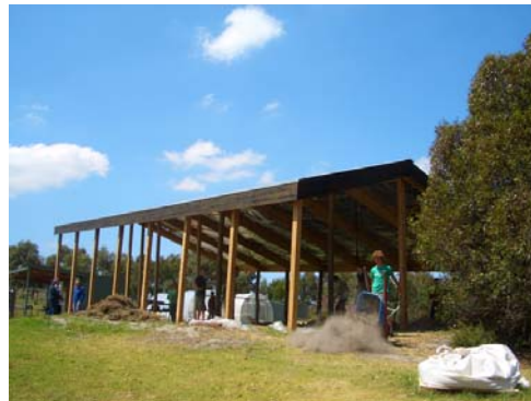
Figure 1 - 3 Students constructing strawbale wall, working under the shelter of the roof & the finished weatherboard clad wall
