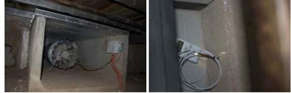
Figure 18 Labyrinth fan (left) & sensor (right) located in rammed earth wall.
